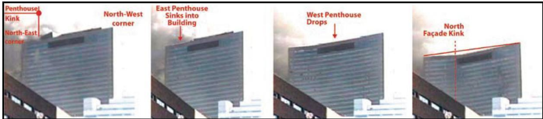
Start of the final collapse sequence (7.7 seconds elapsed). Note that the kink in the east penthouse in the first photo “shifts” towards the middle of the building in the fourth photo, indicating horizontal progression of the collapse.
