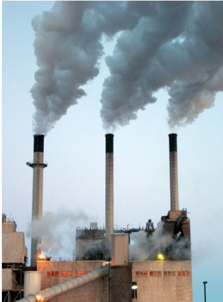
Coal-Burning Power Plant
